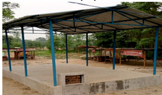
Open pucca shed at Narayanpur Bazar
