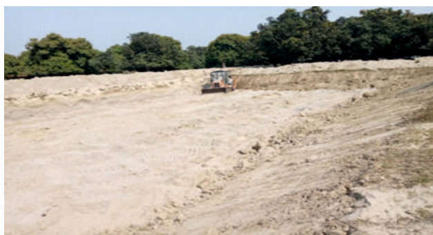
New pond construction
