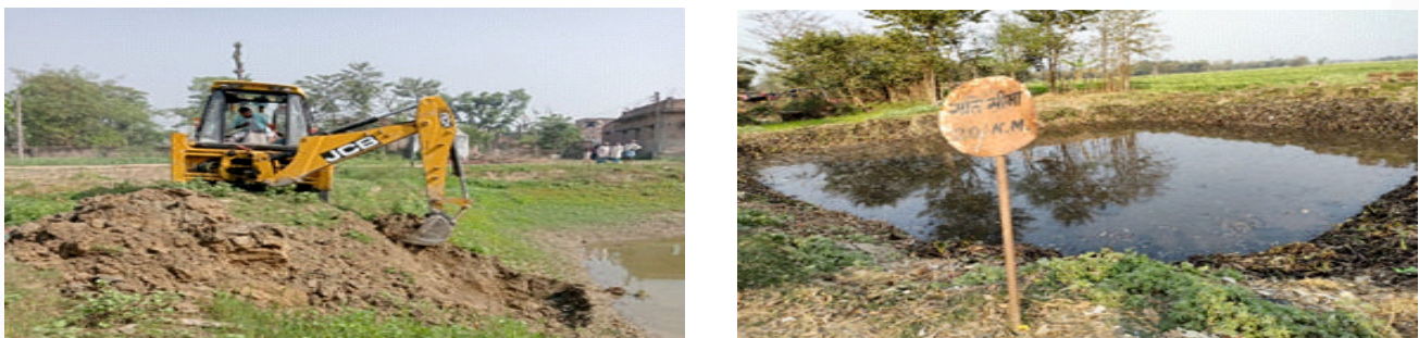
Fig. 27: Reshaping and improving dykes in a community owned pond in Ujheelpur village
