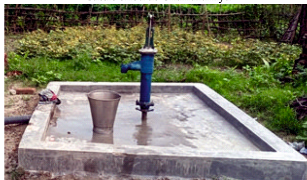
Borewell & handpump at Mahuawa
