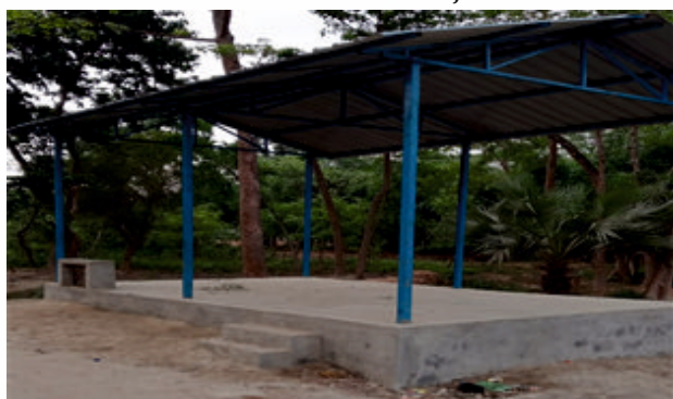
Open pucca shed at Chheni Chhapara
