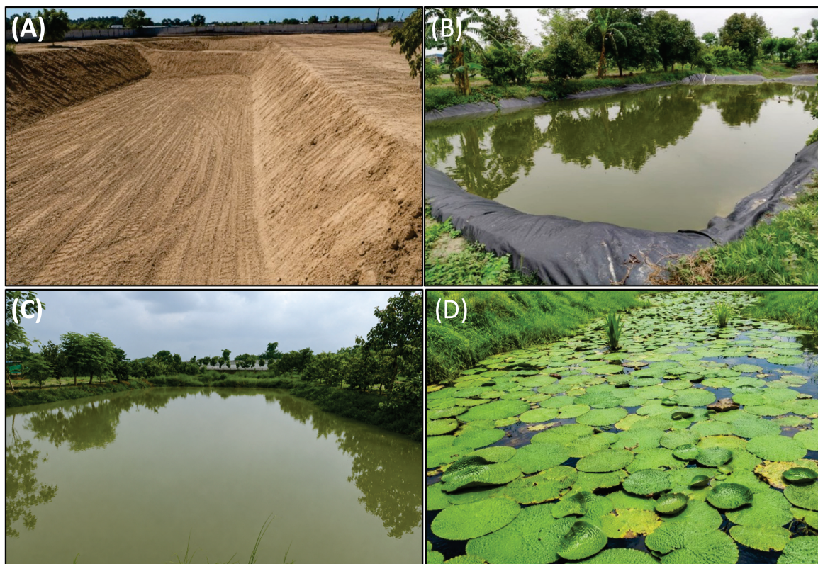
Figure 8.6. Land Shaping for Crop Diversification and Horti-Based IFS project showing (a) initial construction of water harvesting ponds, (b) HDPE-lined pond for efficient water storage, (c) earthen pond utilized for rainwater harvesting, and (d) cultivation of makhana in harvested water. Source: ICAR-MGIFRI
