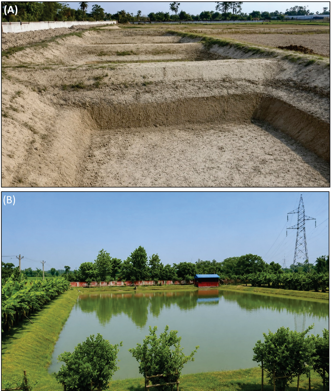
Figure 8.4. Development of the 3,600 m 3 Central Aquaculture Pond under the Fish-Based IFS model: (A) Pond during the initial construction phase; (B) Aerial view of the completed pond at peak water storage. Source: ICAR-MGIFRI
