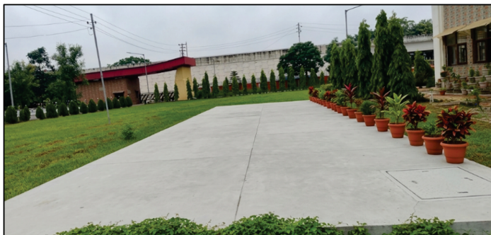
Figure 4.2. Underground Rainwater Storage Tank for long-term storage of harvested rainwater. Source: ICAR-MGIFRI.
