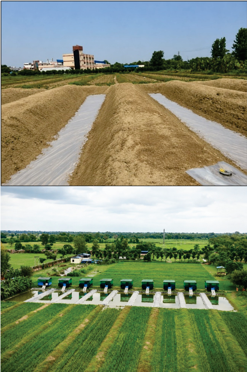
Figure 8.8. Series of HDPE-lined ponds under the Rice–Fish–Duck IFS developed for efficient rainwater harvesting, fish production, and supplemental irrigation in integrated farming. Source: ICAR-MGIFRI
