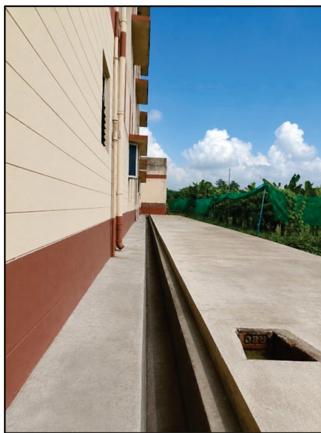
Figure 3.1. Roof gutter used for collecting and conveying rainwater from rooftop catchments. Source: ICAR-MGIFRI.
