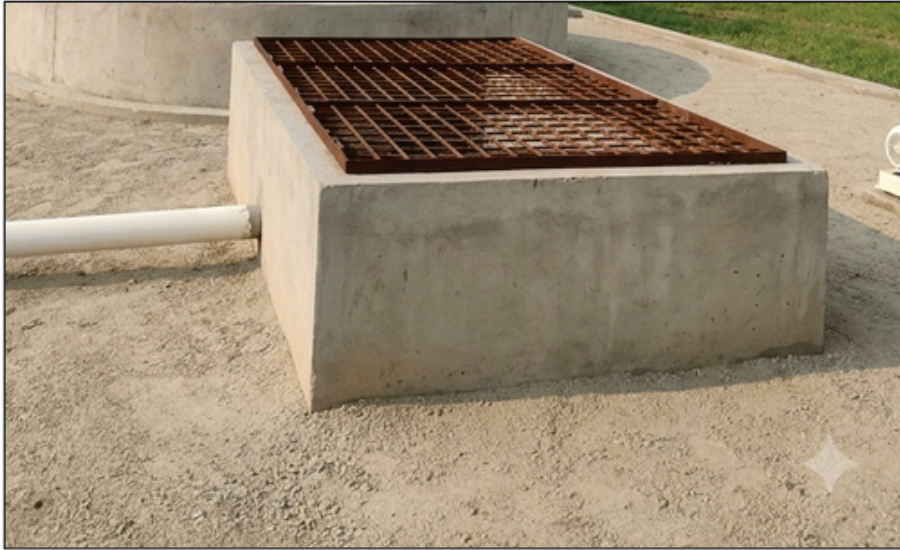
Figure 3.8. Settlement Tank for sedimentation and removal of suspended particles. Source: ICAR–MGIFRI.
