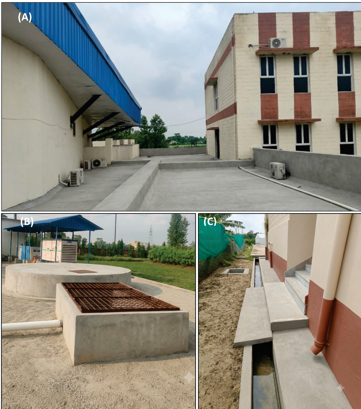
Figure 8.2. Auditorium rooftop rainwater harvesting and storage system showing (A) rooftop catchment, (B) PVC gutters and downpipes, and (C) storage tank at ICAR-MGIFRI, Piprakothi. Source: ICAR-MGIFRI
