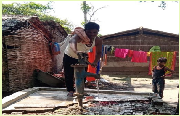
Borewell & handpump at Naraha
