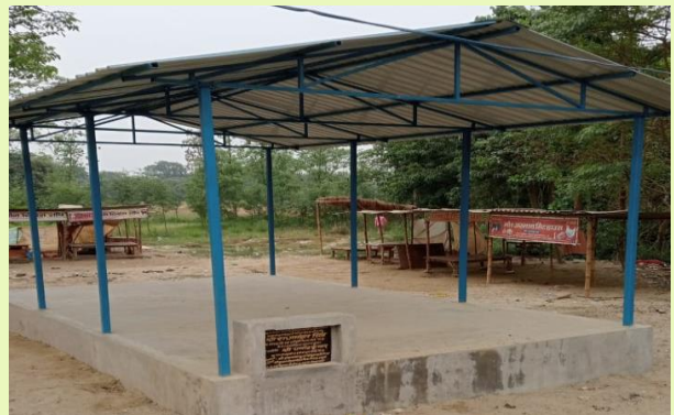
Open pucca shed at Narayanpur Bazar
