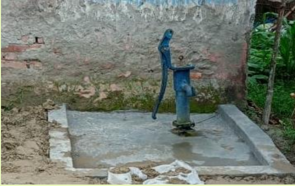
Borewell & handpump at Fursatpur
