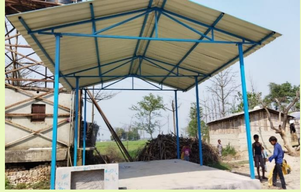
Open pucca shed at Hanuman Nagar
