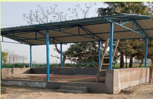
Open pucca shed at Hasanpur
