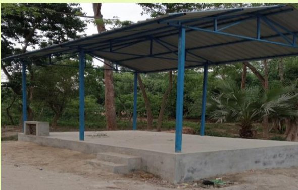
Open pucca shed at Chheni Chhapara
